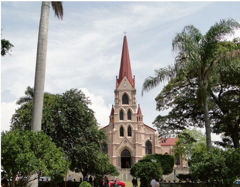
Fig. 128.4 Costa Rican Lesmes Jiménez Bonnefil, a mining engineer designed the neogothic Church of La Merced in San José in 1894 (Photo by Martín Checa-Artasu)
